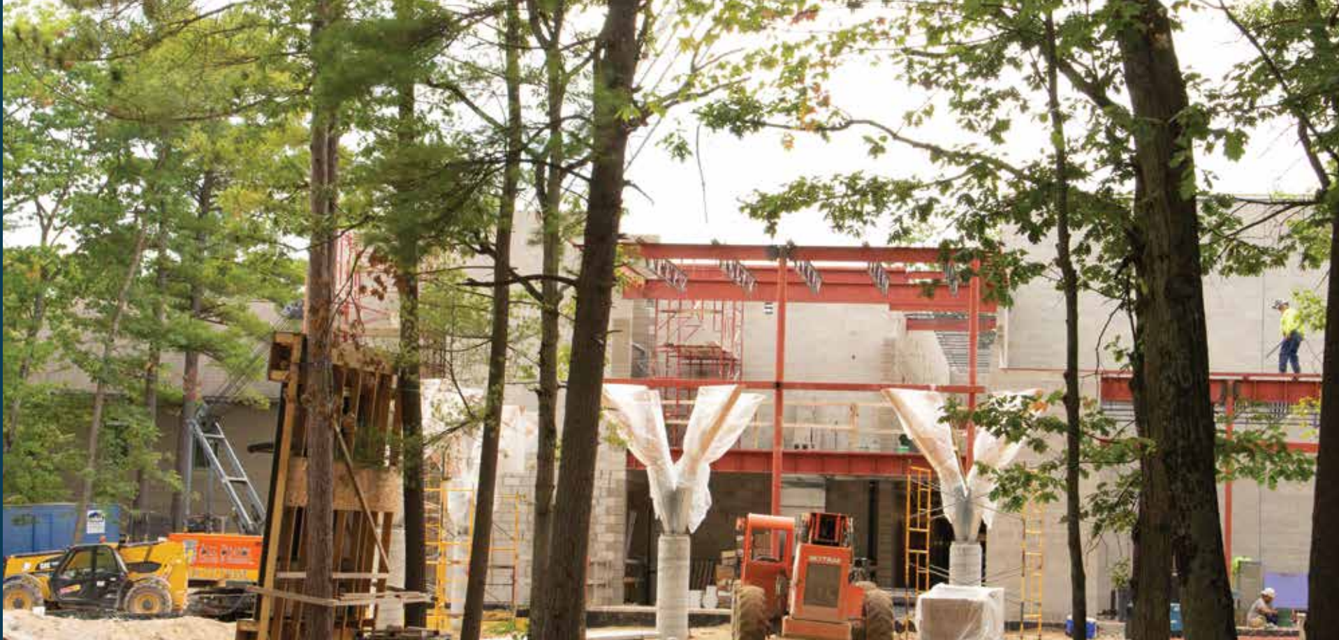
Construction of the new Music Building is set for completion spring 2019
